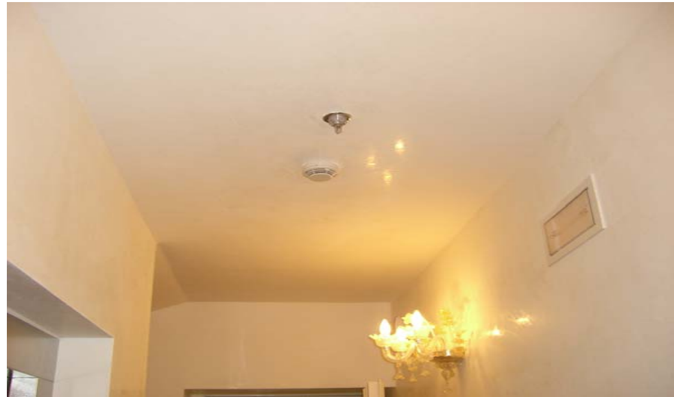
Ugello Water Mist EI-FOG automatico
